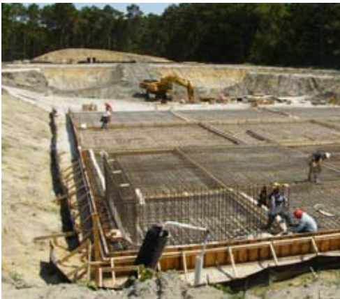
Check out the progress on the Town's new WWTTP!!!!
