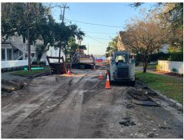
water, drinking water, and sewer) systems on the 100 block of Orange Street. UNC-IMS water quality experts have seen a strong signal of toxins at the storm water outfall at the end of Orange Street, and these repairs on the 100 block should mitigate some of the sources of this pollution. This project also includes large sections of pervious surface on the street surface as another way to reduce storm water effects.
