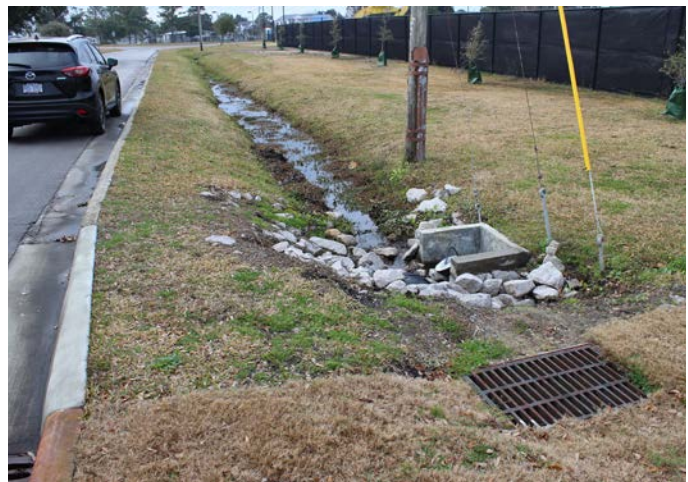
Stormwater drainage area
