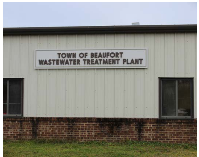
Town Wastewater Treatment Plant
