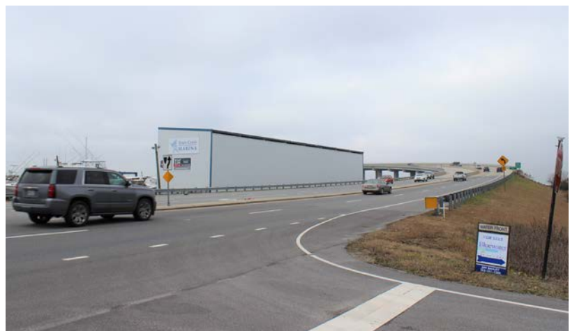
Highway 70 bridge over Gallant's Channel
