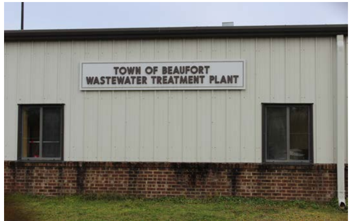
Town of Beaufort Wastewater Treatment Plant
