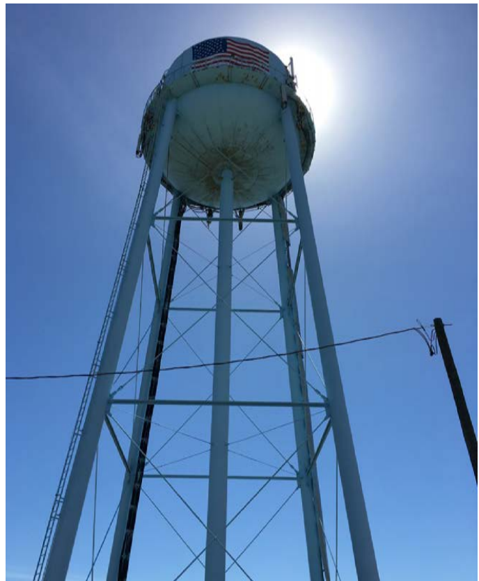
Beaufort Water Tower
