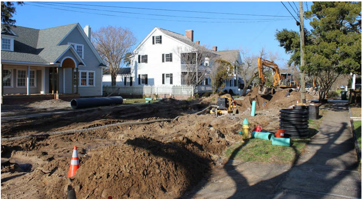
The Town is actively engaged in infrastructure upgrades and maintenance.
