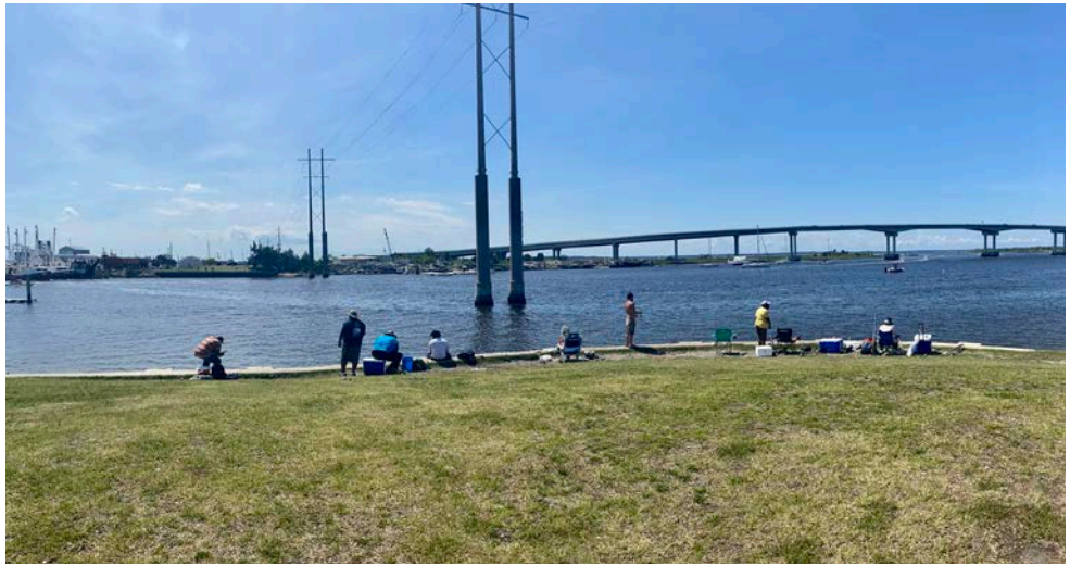
Gallants Channel Bridge
